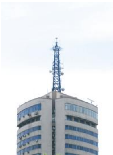
Nanjing VTS center and Daqiao adar station
