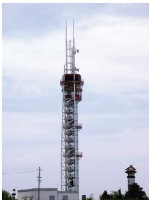
Liuwei estuary microwave relay station
