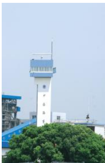
Yizheng radar station
