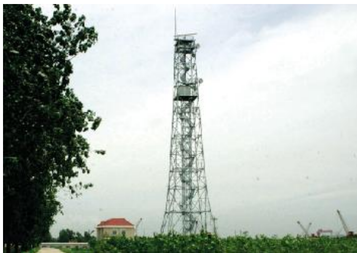
Jiaogang radar station
