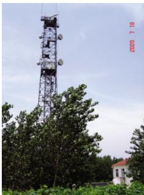
Fudewei radar station
