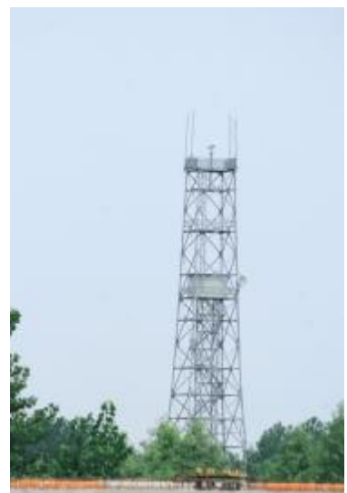
Tianhekou radar station
